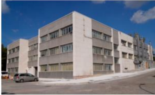
Fig. 5: South-west view of the building Before renovation.
