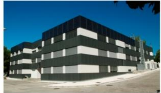
Fig. 6: South-west view of the building After renovation.
